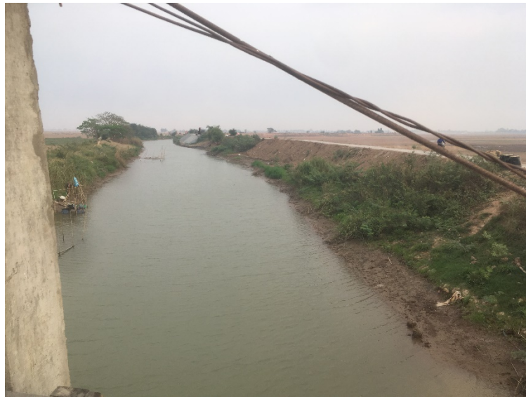
Figure 6: View onto hard dyke. Far away one can see the reconstruction work
