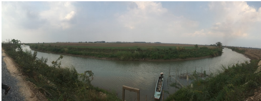
Figure 5: View from hard dyke onto soft dyke and fields that get flooded each year. In the lower middle, left of the boat one can see a pump. On the far-right side one can see the cemented part of the hard dyke.
