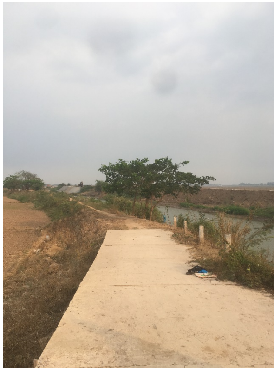
Figure 7: One can see the soft dyke and beginnings of cementation which leads to nowhere.
